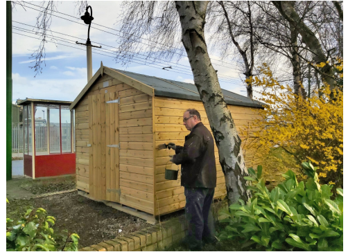
Mike Spilling applies preservative to the new cycle shop shed.
