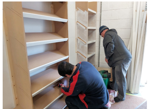
Mark Boulton and his father installing new shelving in the Trolleyshop.
