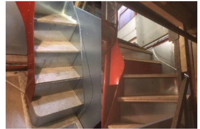
Above: The staircase rebuilt – the original inner stringer and one riser were salvaged and repaired but other parts had to be fabricated using old bits as a pattern
