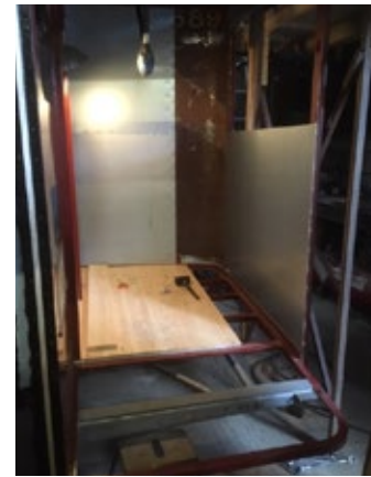
Above: Rear platform area under reconstruction
