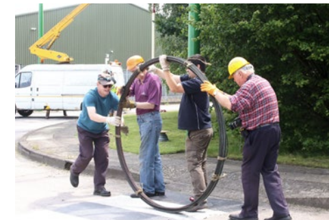
Ian Brown, Bruce Lake, Mark Boulton and Bob Ashton roll the running wire into place while behind them the cherry picker and (out of sight) the Bradford tower wagon are being used by Andy and Norman. (DC)
