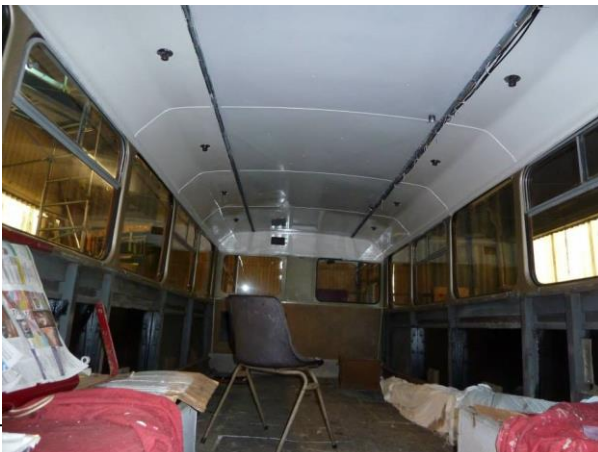
Below: The newly repainted lower ceiling (1 May)
